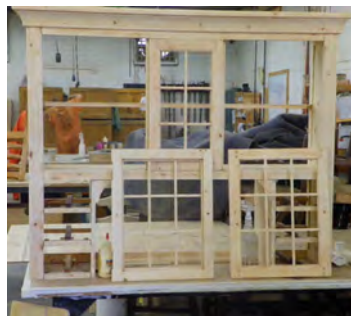
Trusses and frame fabrication in the new Red Rock facility in Eloy will benefit from the experienced craftsmen who learned their skills in the various ACI shops.
