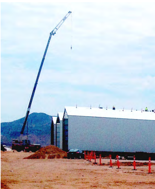
Hickman's new Tonopah facility under construction
