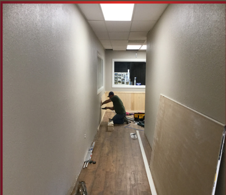
Danny Jones installs a chair rail in the new visitor center.
